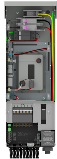
Figure 7 Chamber wiring
