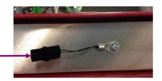
Kit provides an alarm when a GPS4848 Distributed Architecture Inter-bay bus temperature is high. A probe should be located off framing or racking above the initial cabinet to provide ambient temperature. A kit should be applied to each -48V inter-bay bus: 1 kit per supplemental cabinet. Probe mounts to an inter-bay bus and connects to 221F or 223T RPM module.
