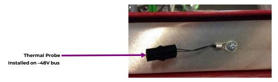
Kit provides an alarm when a GPS4848 Distributed Architecture Inter-bay bus temperature is high. A probe should be located off framing or racking above the initial cabinet to provide ambient temperature. A kit should be applied to each –48V inter-bay bus: 1 kit per supplemental cabinet. Probe mounts to an inter-bay bus and connects to 221F or 223T RPM module.
