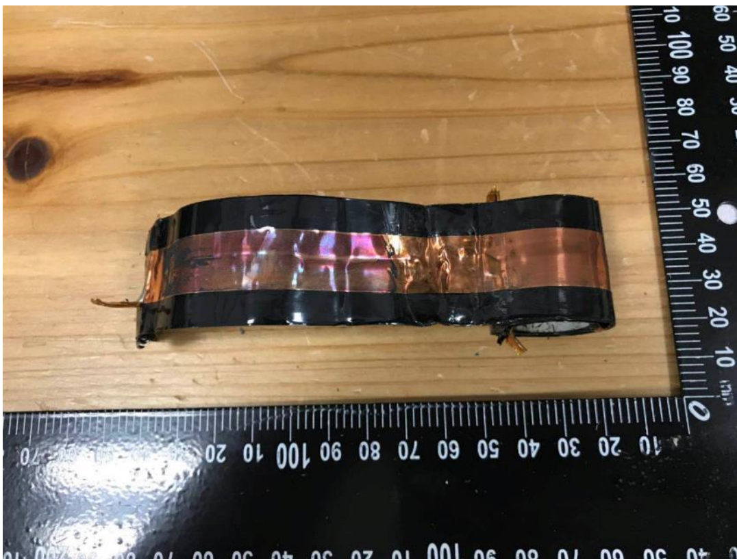
Picture 22 – Transformer T300
