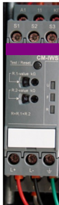
Figure 34 Ground Fault Indicator
