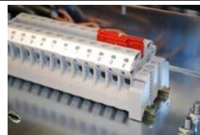
AC per three rectifiers (2 jumpers between 3 blocks)
